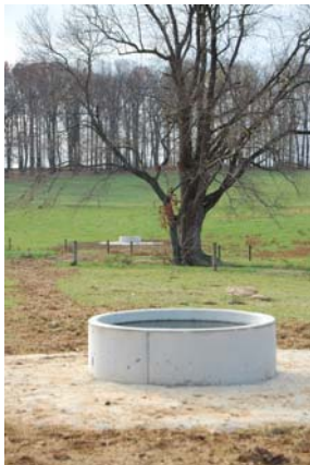
Gravity-fed watering trough, providing clean drinking water for live-stock.
