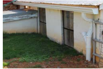
Roof runoff structures divert clean water and prevent erosion.
