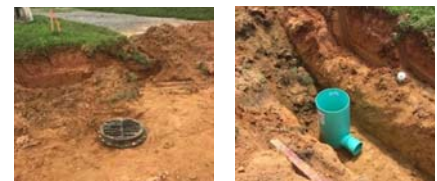
Components of a grade stabilization structure: grate (top left), drop pipe (top right), and pipeline (right).
