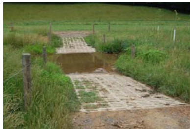
Ford stream crossing made of precast concrete panels.
